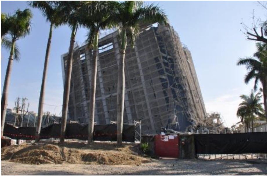
Figure 3. Tilt failure of buildings induced by tectonic earthquakes (Hsu and Ho, 2016).
