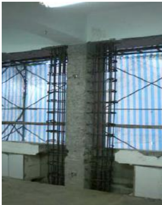
Figure 8. RC wing wall reinforcement method (Zhong, et al., 2009).
