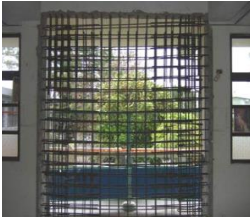
Figure 9. RC shear wall reinforcement method (Zhong, et al., 2009).
