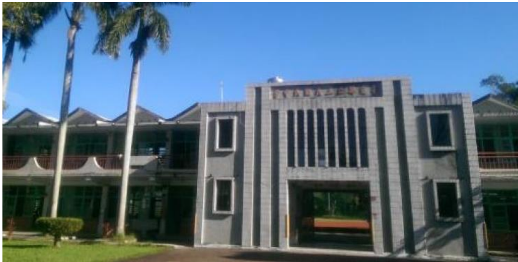
Figure 11. Sanmin Junior High School, Hualien, which remained stable during the 0206 Hualien earthquake in 2018 (Standard School Building of Hualien Sanmin Junior High School, 2016).
