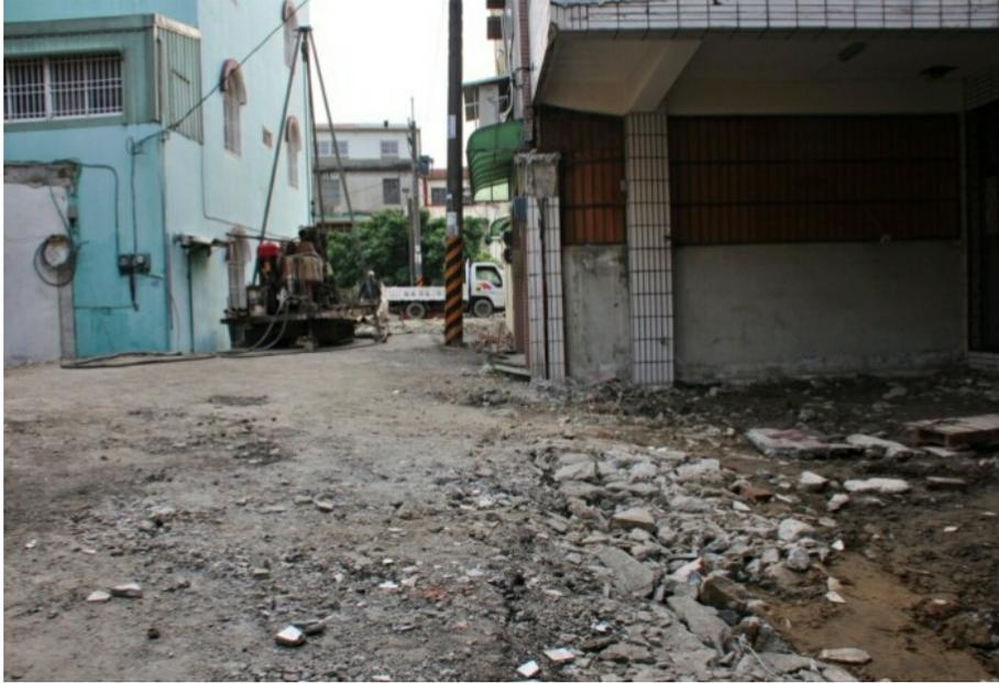
Figure 10. In-situ drilling operations performed by traditional scholars in a non-shear band area in Tainan where liquefaction will not in fact occur.
