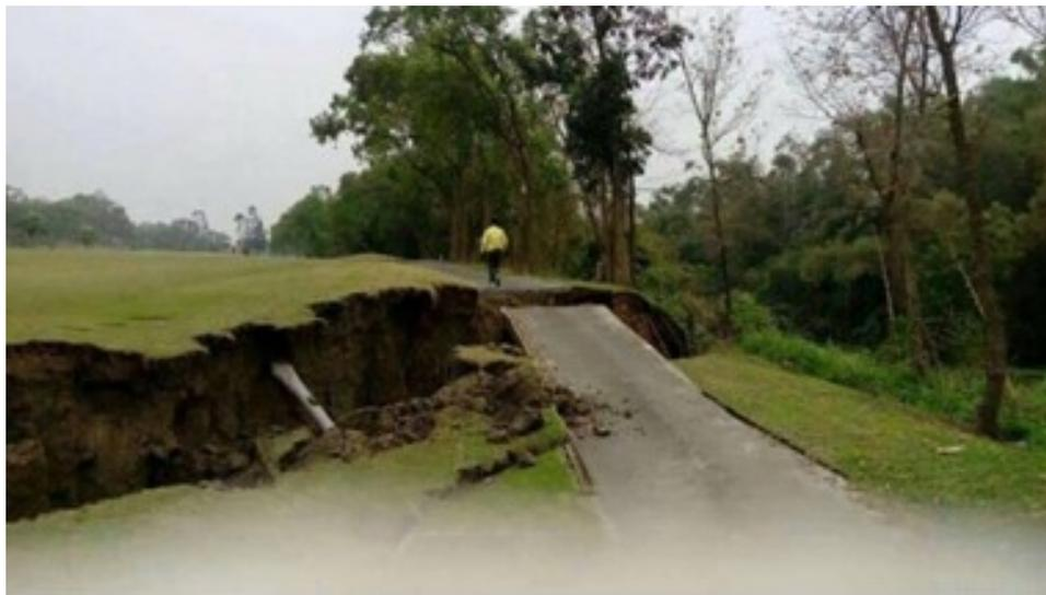
Figure 2. Striped soil liquefaction took place during the Meinong Earthquake (Liberty Time Net, 2016)
