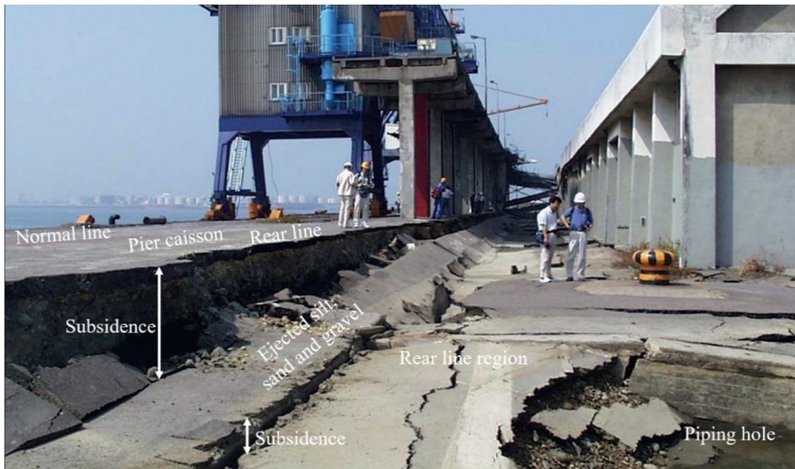
Figure 11. Three different types of seismic failure that occurred in the rear line region of the caisson piers at Taichung Port during the 921 Jiji earthquake (Hsu, 2022).
